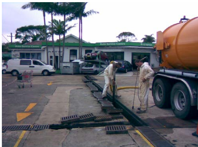
Figure 2.0 Harris Farm drain clearing was carried out January 2014.
