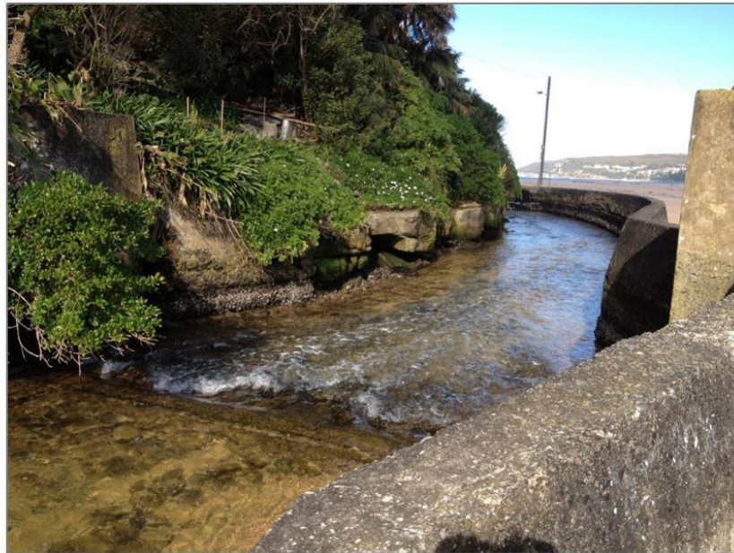
Figure 6-4 Manly Lagoon concrete entrance channel
