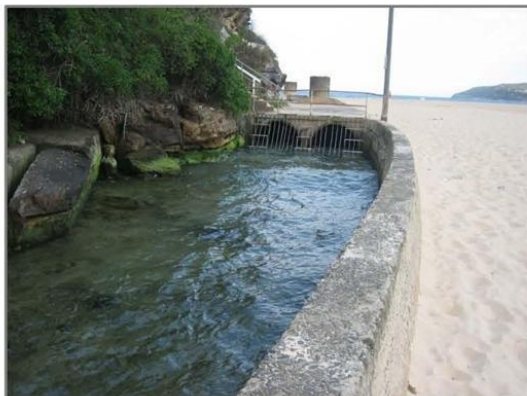
Low-flow pipes at channel entrance
