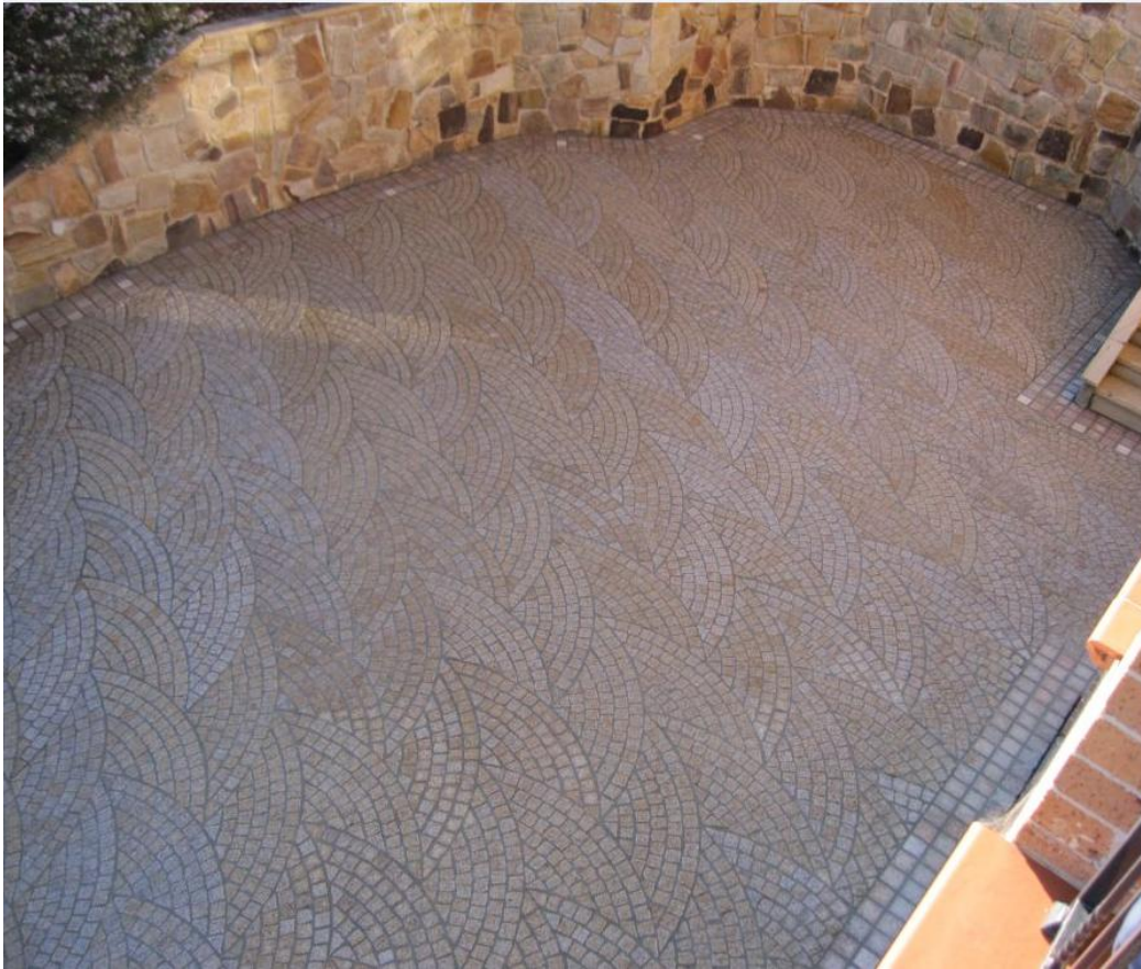
Shell, scale or wave fan shaped pattern of exfoliated granite paving proposed for public space at intersection of Bower Lane and Marine Pde
