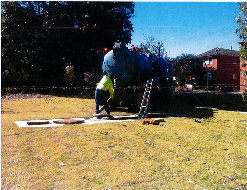
Fig. 7 GPT Cleaning Balgowlah Road by MGC.
