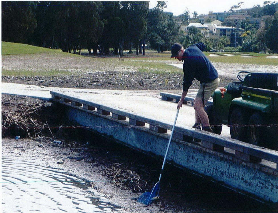
Fig. 5 Rubbish removal at bridges
