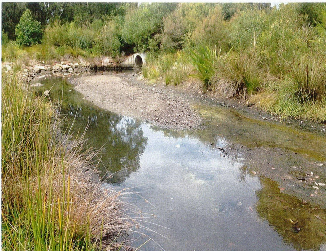
Fig. 8 Sediment and Organic Matter accumulation from Fairlight Hill catchment
