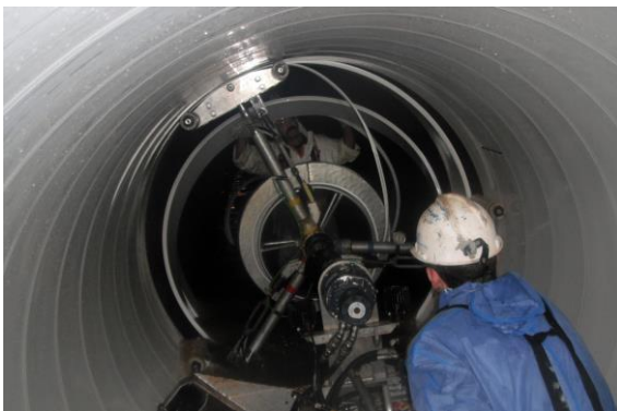
Installing the new structural liner
