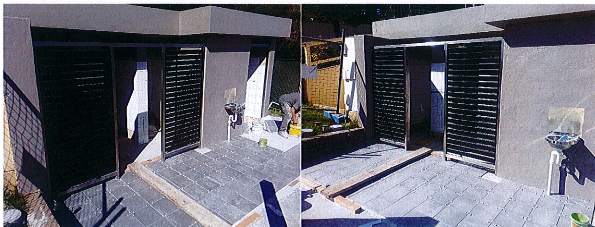
Progress photos 02 Oct 2014
