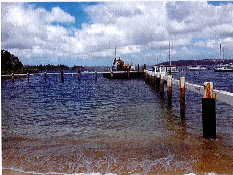
Figure 1. Little Manly saltwater pool during installation of sea horse friendly netting.
