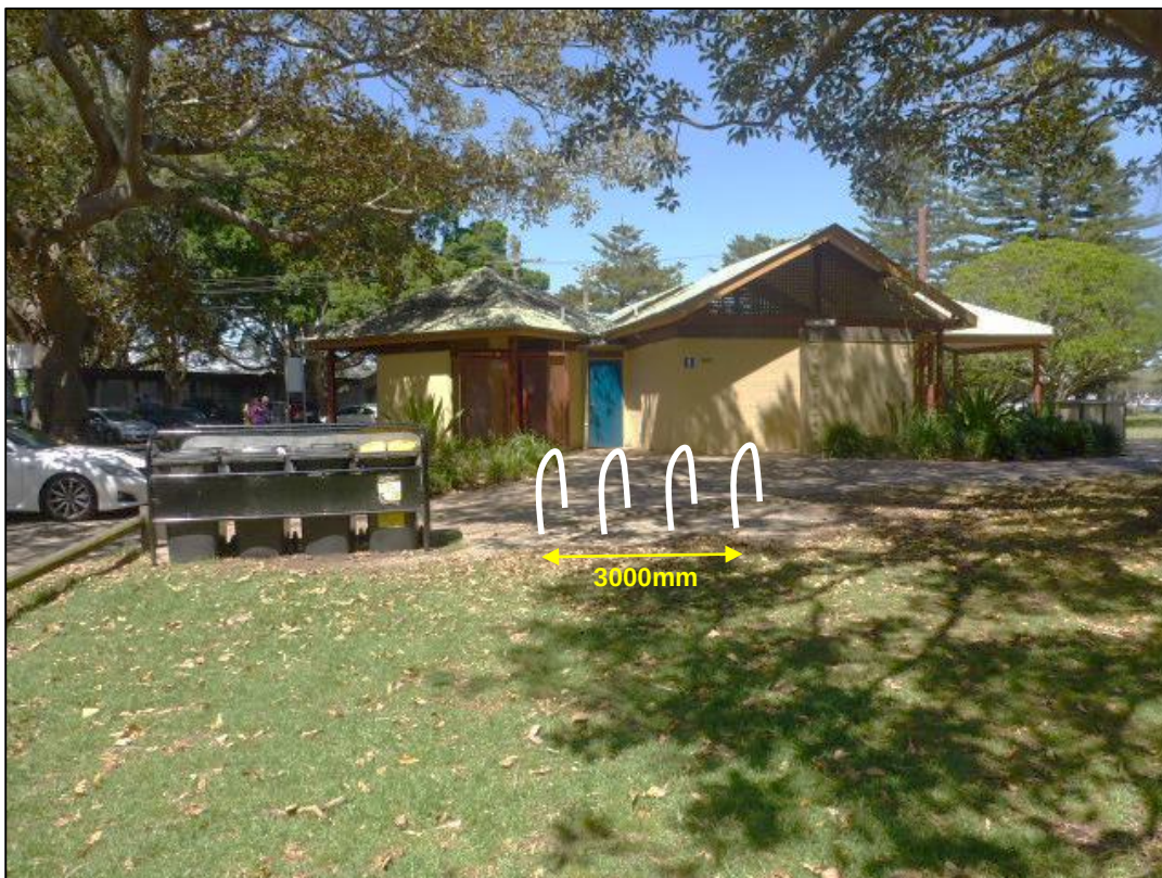
Figure 2: Clontarf Reserve – Installation of four (4) U-rails
