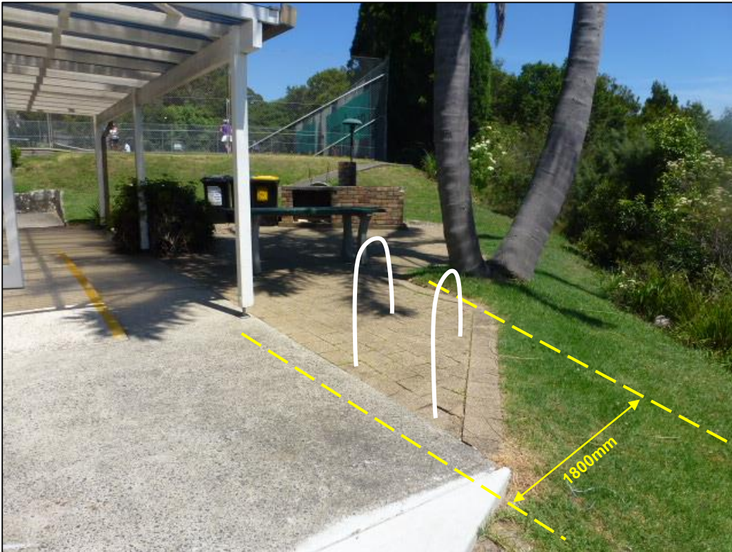
Figure 3: Bareena Park – Installation of two (2) U-rails
