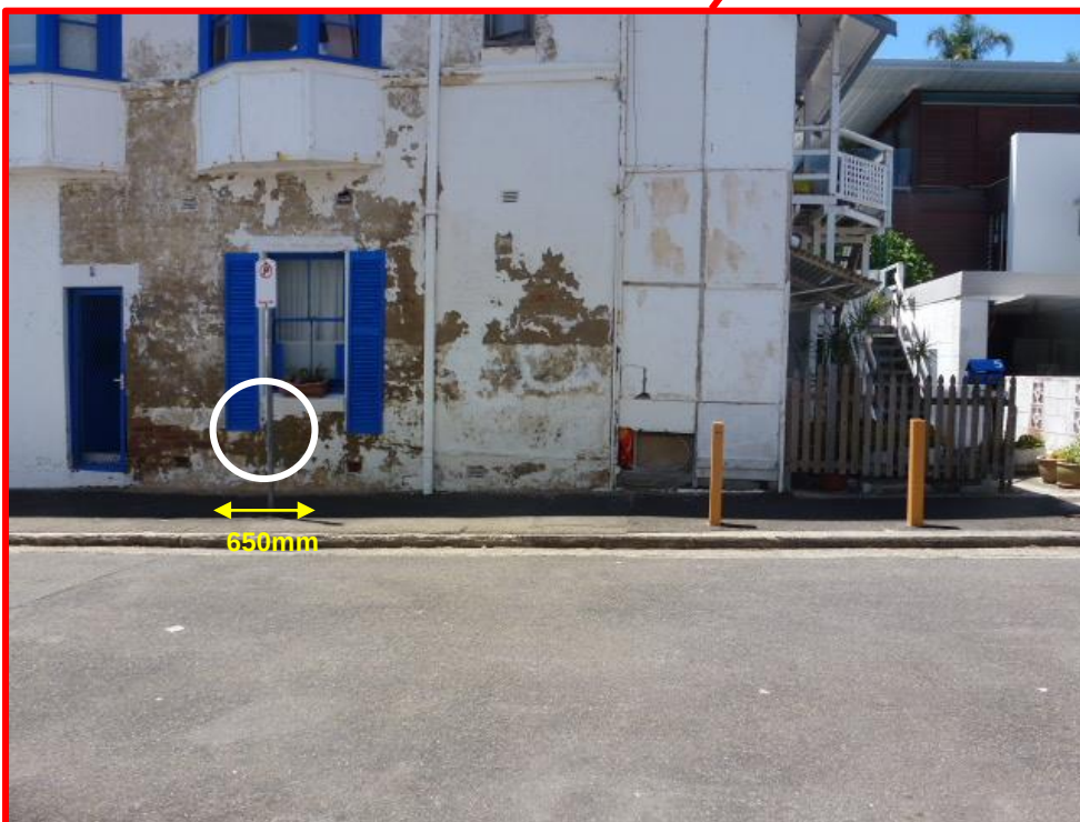
Figure 5: Bower Lane (Shelly Beach) – Installation of one (1) post mounted bike rail
