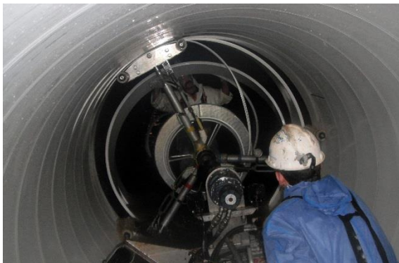
Installing the new structural liner
